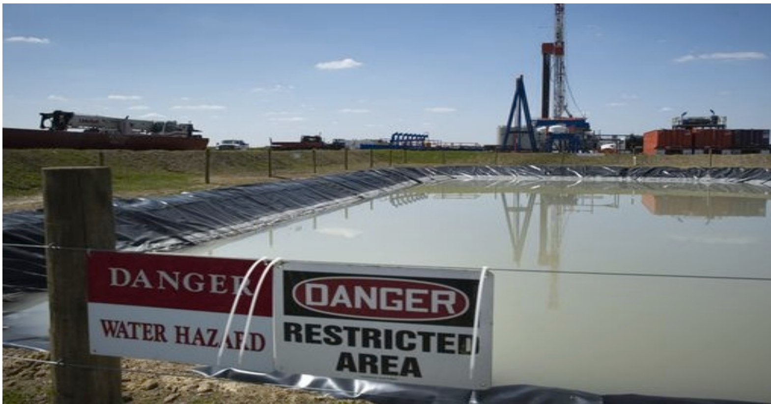
Figure 11: Industrial effluent pond holds contaminated water on the surface near a fracking well.
